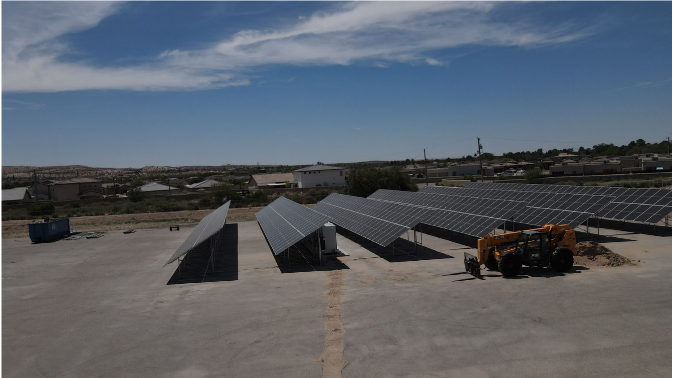
Solar Array progress picture
