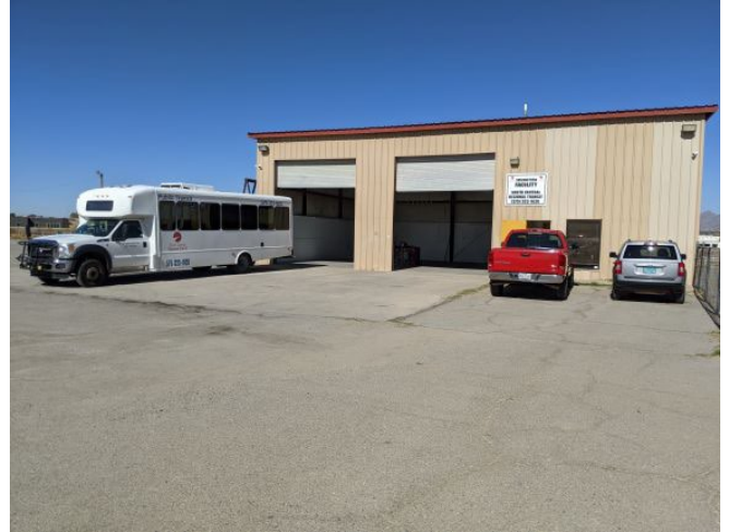
Sunland Park Transit Facility
